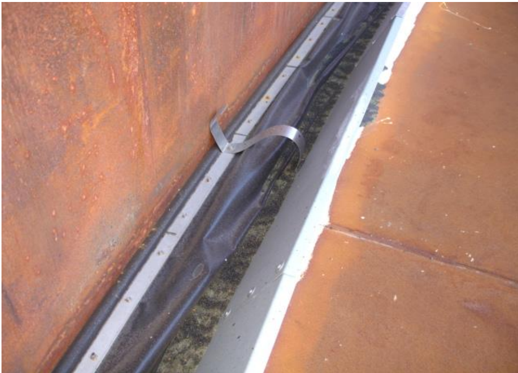
Typical shunt and secondary seal
