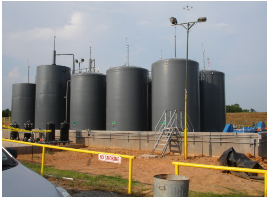
Typical production/disposal tank battery
