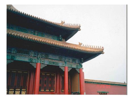
The ancient Chinese recognized that lightning was most likely to attach to corners and edges of a structure. If you look at the roof an old Chinese building such as one found in the Forbidden City, you will notice a parade of small, fearsome looking figurines arranged along the edges. The purpose of these figurines was to frighten away lightning. They unintentionally comprised the lightning strike interception component of the first lightning protection systems.
