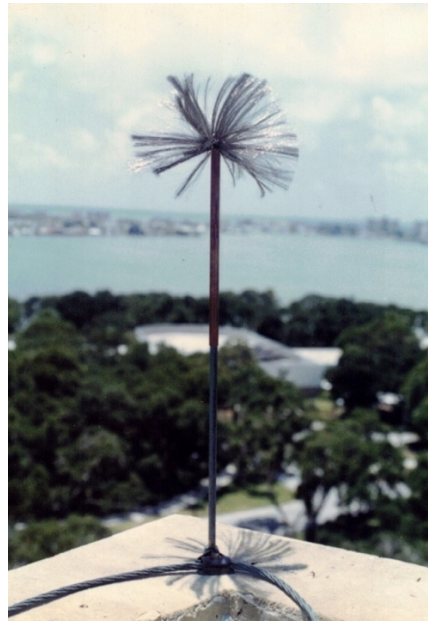
Early Slip-Over Ultra Sharp Point Air Terminal
