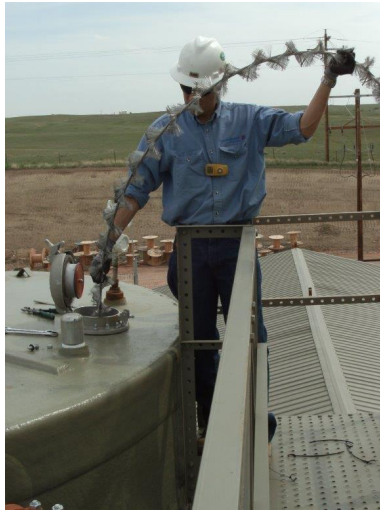
Installing ITSD through a production tank thief hatch
