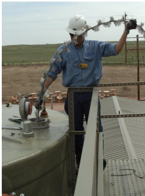
in-tank static drain in production tank
