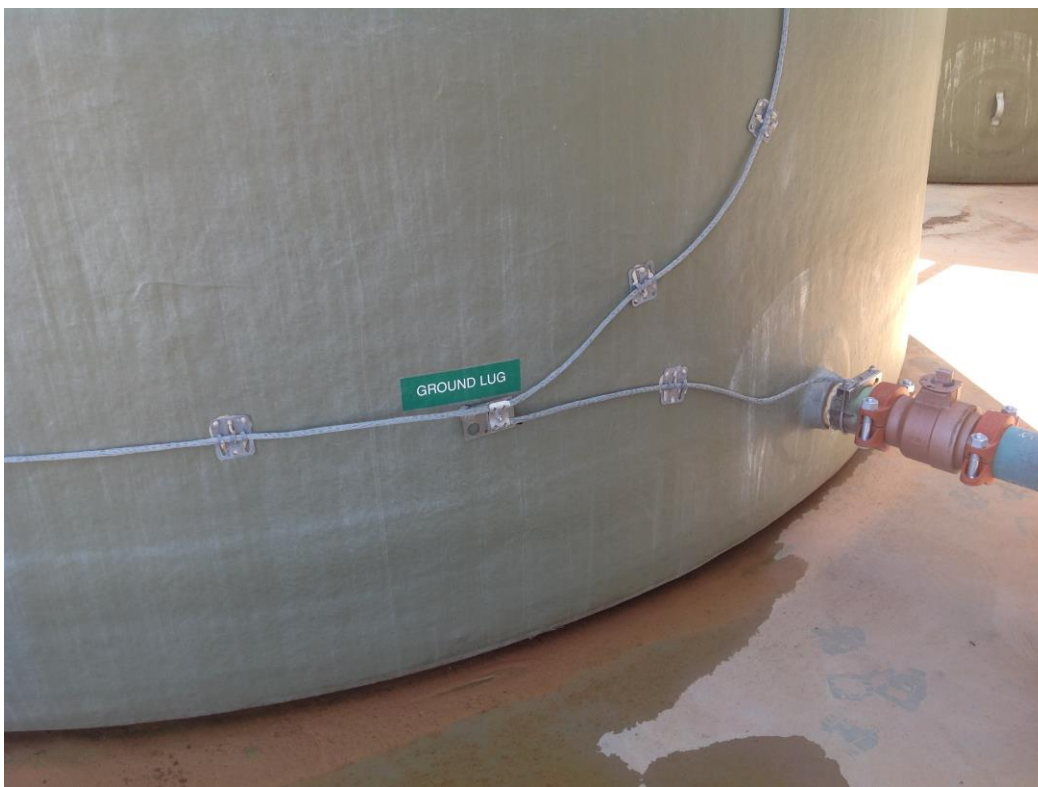
tank-base piping and carbon veil bonding
