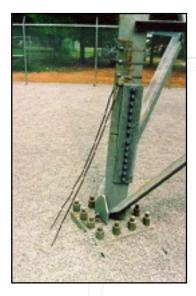
connecting them with conductors, bringing them to the same electrical potential. The primary reason for bonding is personnel safety, so someone touching two pieces of equipment at the same time does not receive a shock by
