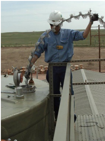
Installing ITSD through production tank thief hatch
