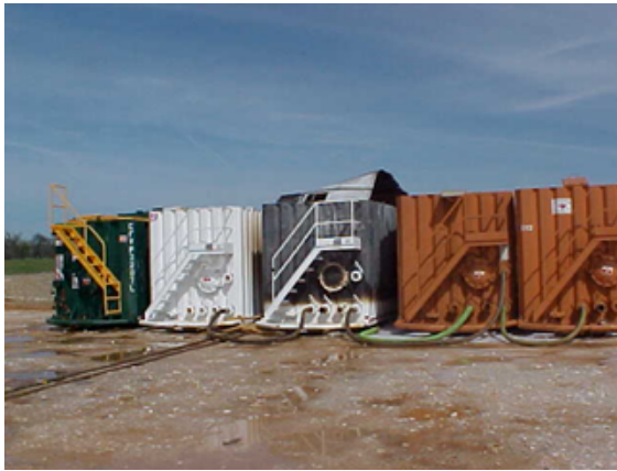
Damage to closed flowback tank caused by static ignition
