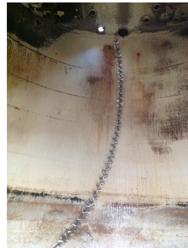
ITSD inside tank
